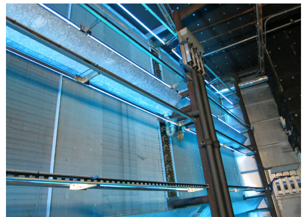
A large Fresh-Aire UV surface UVGI installation
